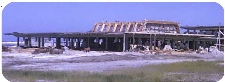
Sheen B Building under construction in 1963
