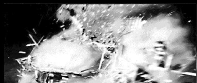
A wood-frame house exposed to a nucear blast at the Nevada Test Sie on March 17, 1953. The house is 1,100 meters from ground zero. http://atomicarchive.com
